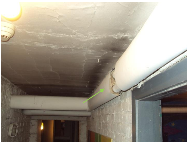
Photo 3 Cave , couloir, calorifuge
