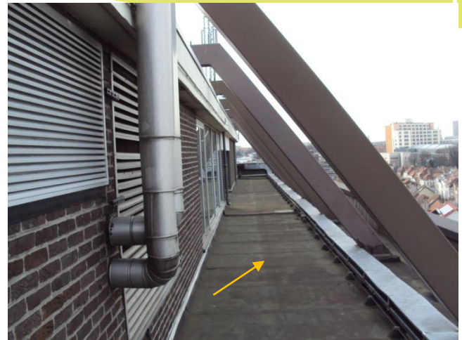
Photo 6 Zone administrative, toiture
